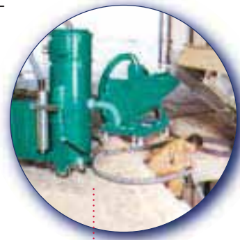
Cleaning of debris from discharge pits.
